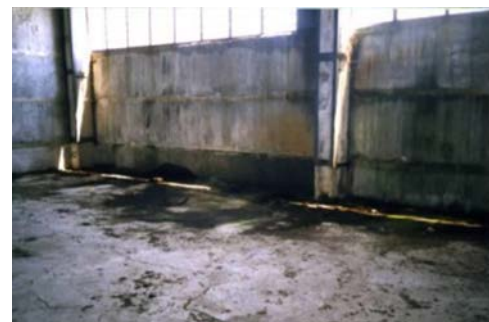
6 th step – Site's decontamination
