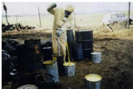
3 rd step – Treatment and solidification
